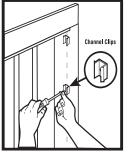
or a 3/32" drill bit) and install the channel clips loosely, using six of the 1" roundhead screws. Align the clips vertically and fully secure the screws. Press the door anchor panel onto them until it snaps into place.
