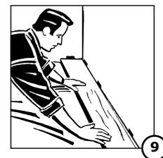
2. An expansion joint of around the thickness of the floor should be installed all around the floor. Place a spacer block at every 40 cm **(see 10)**. Remove them 24 hours after the floor has been laid.
